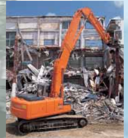
ZAXIS210LCK (High Lift + Backhoe)
