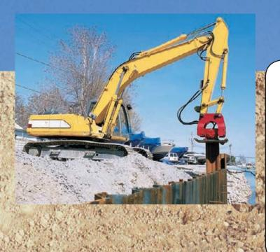
Allied's continuous product improvement has now made a highly successful product — the Ho-Pac® — even better with the Model 300B, Model 500B, Model 1000B, Model 1600 and Model 2300. The all-new extreme Ho-Pacs now deliver more impact energy, an errorless four-function valve, a variety of mounting configurations and maintenance-free sealed bearing or oil splash bearing lubrication.
